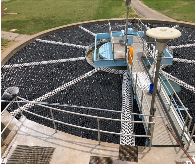
Shade balls deployed on a water treatment clarifier
